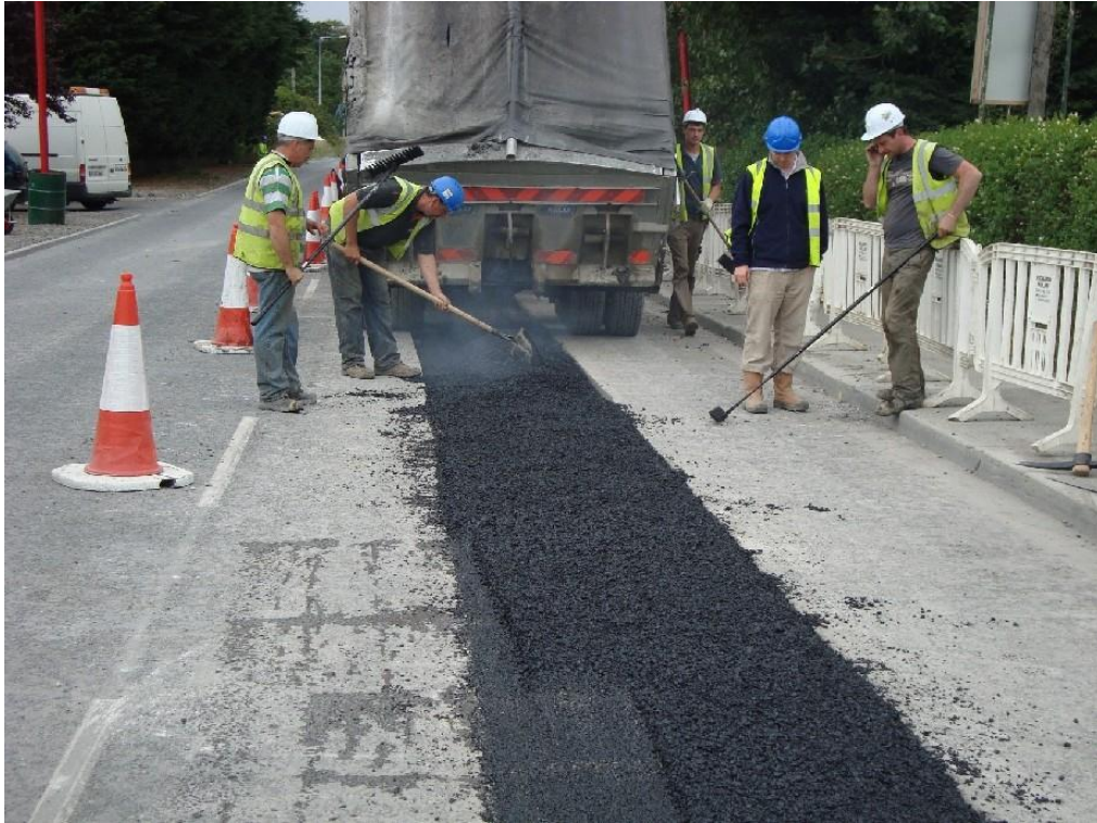
Plate 2 : Reinstatement of road surface over trench
