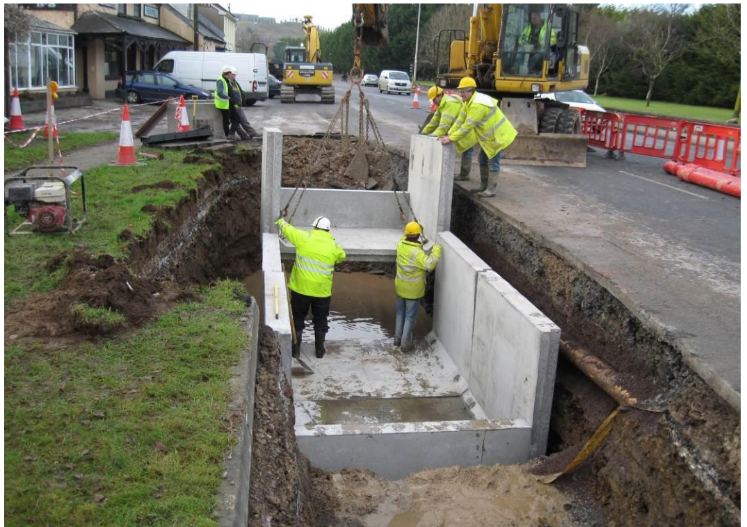
Plate 5 : Typical joint bay under construction (pre-cast)
