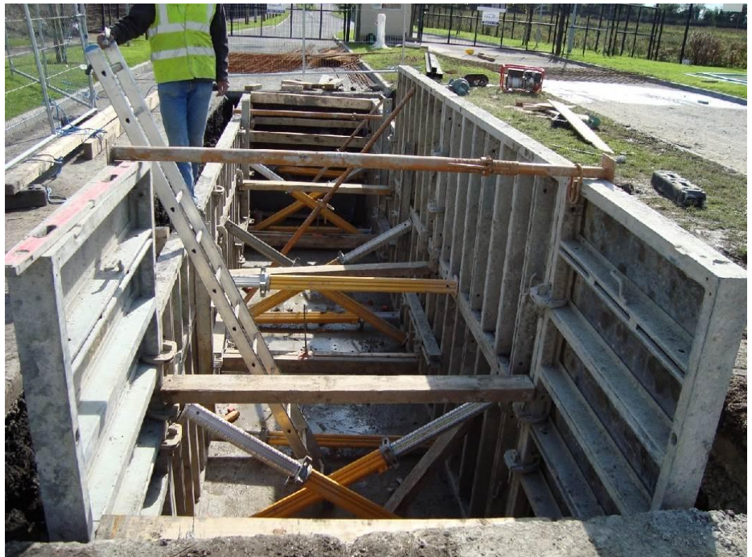
Plate 3 : Typical joint bay under construction (in-situ)
