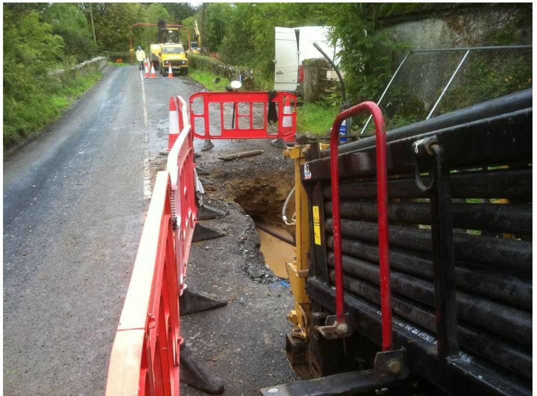
Plate 11: Typical HDD site on local road (Bridge parapet walls visible)
