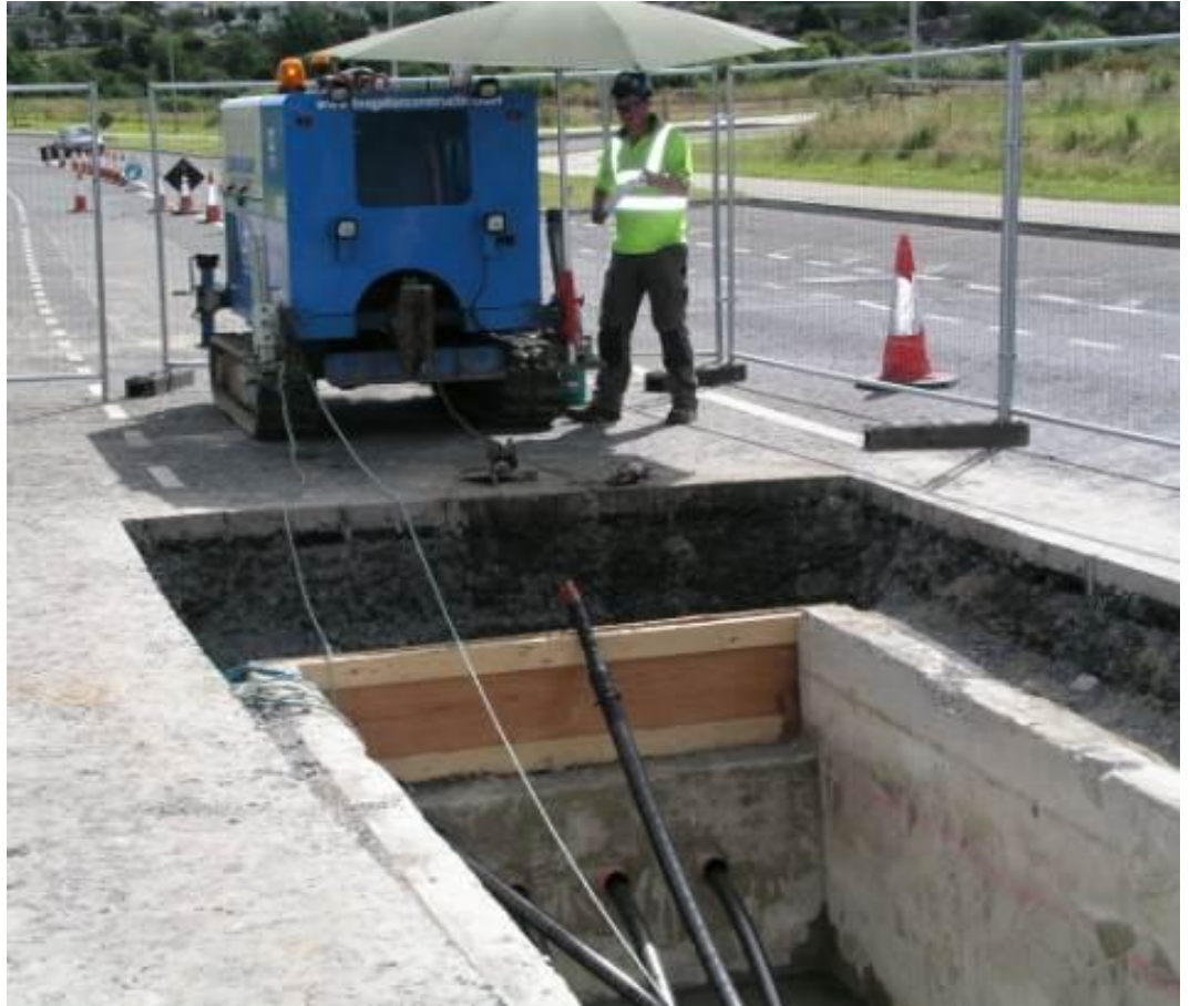
Plate 8 : HV cable pulling procedure (Typical pulling winch set-up)
