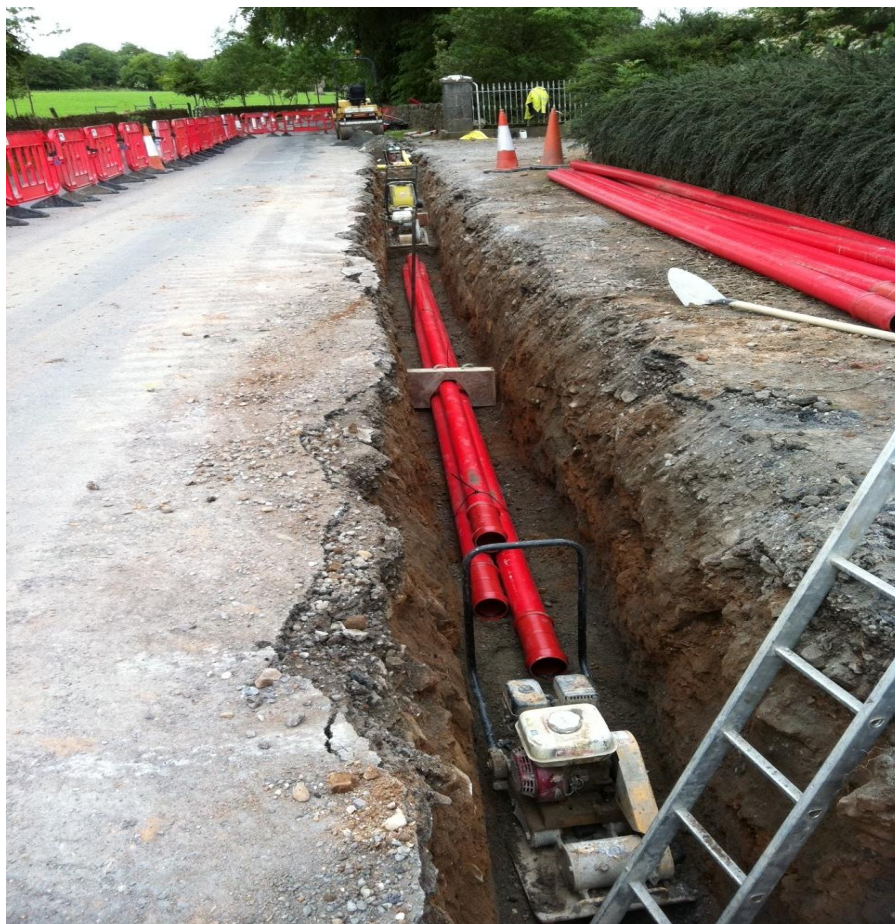
Plate 1 : Typical 110 kV cross section
