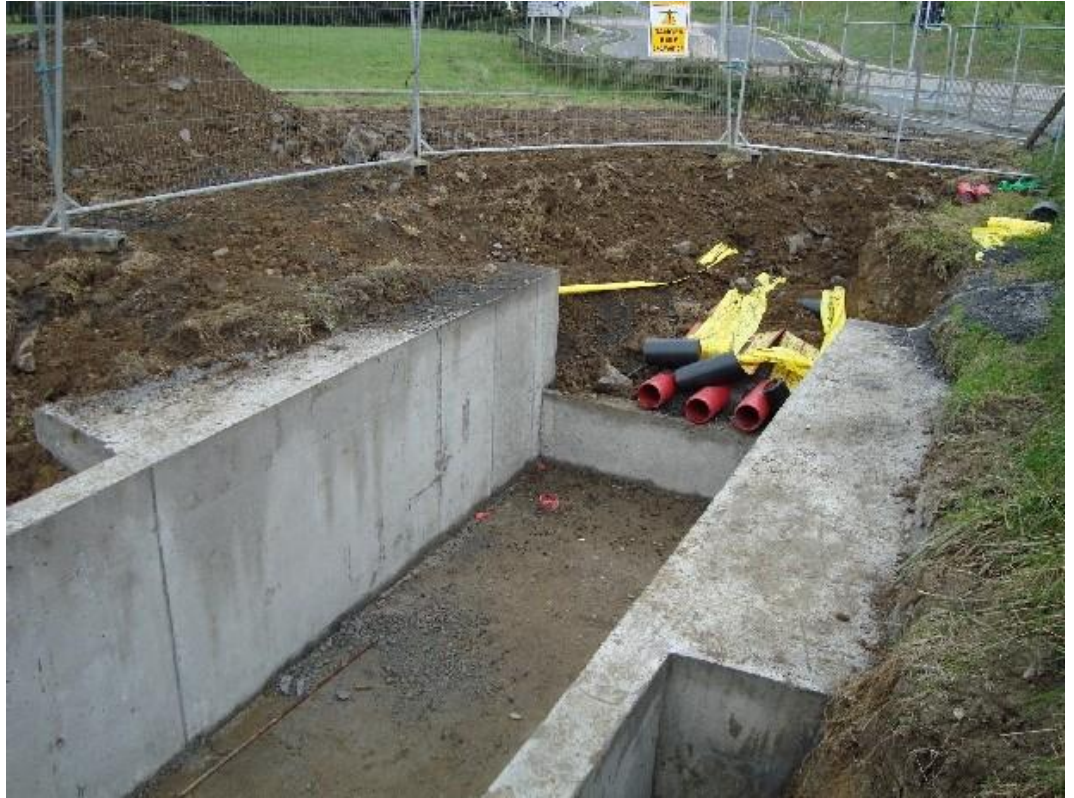
Plate 4 : Completed joint bay prior to cable installation (in-situ)
