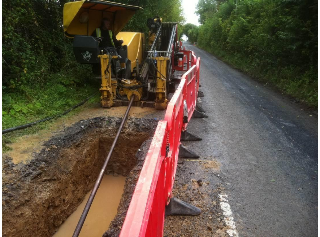
Plate 10: HDD rig set up on regional road.
