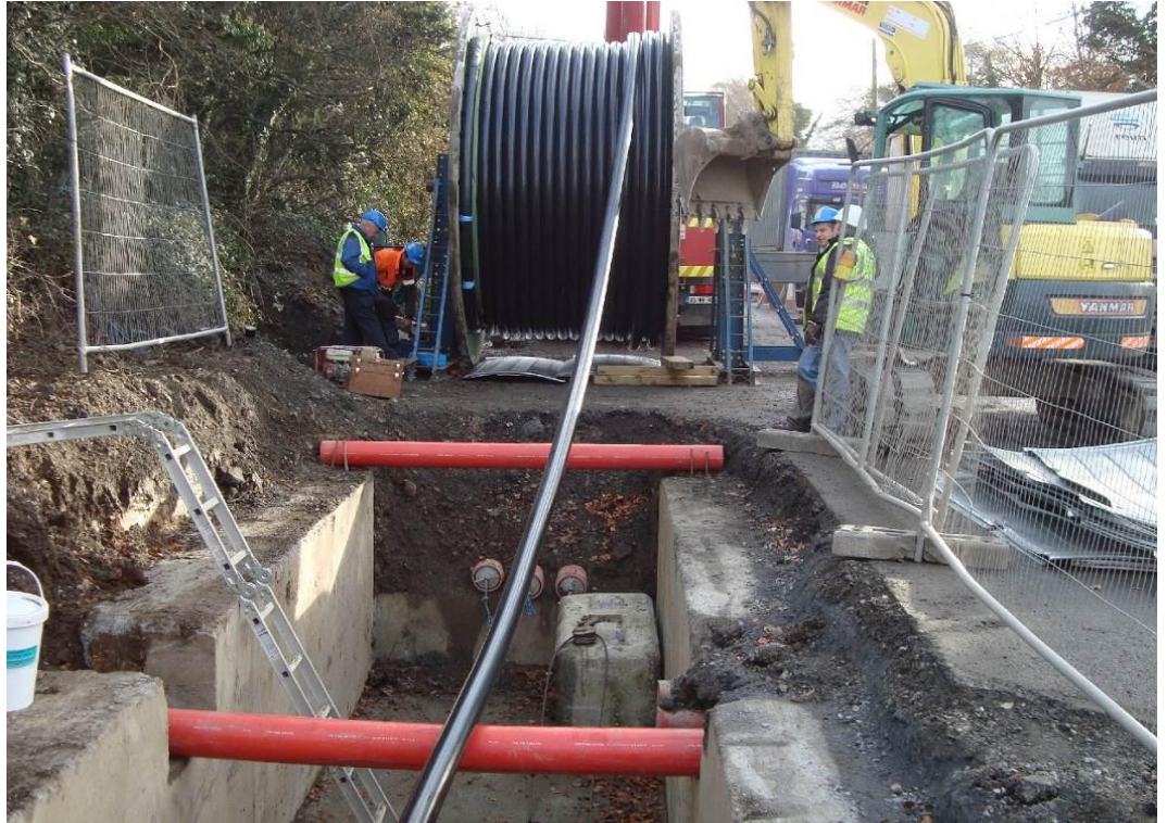
Plate 6 : HV cable pulling procedure (Typical drum set-up)
